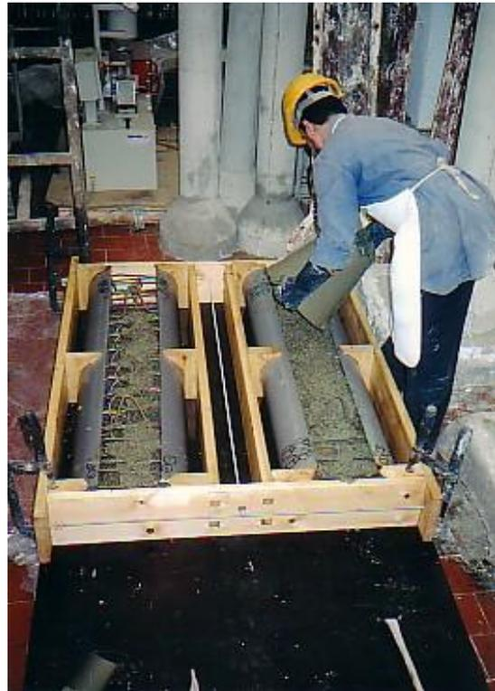
**Photo 3. Casting of Concrete Columns**
